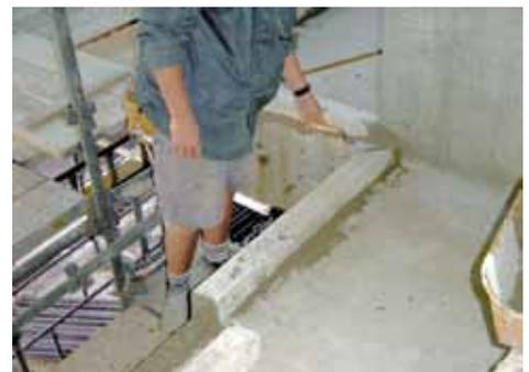
Ultralintel being bonded to create the hob.
