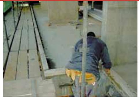
Hob being bonded to slab edge.
