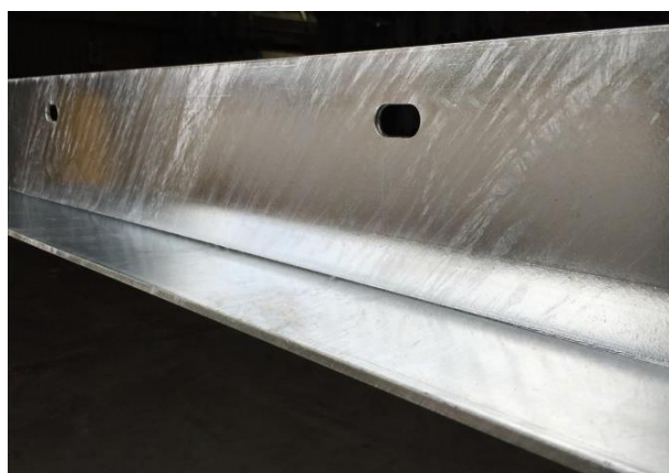
Slots in vertical leg - view of internal face
